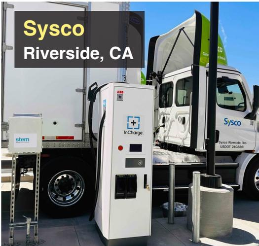
As one of the first of its kind in the world, Sysco's Riverside Electric Vehicle Hub will include 40 dual port DC fast-charging stations in support of 40 Electric, Class-8 vehicles, and 40 electric refrigerated trailers. The Hub will also include 4 MWh of battery storage and increased solar power generation by an additional 1.5 MW to accommodate the energy demands of its growing fleet.
