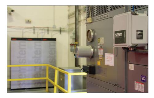
In March of 2014, Stem installed a 54 kW energy storage system, which uses real-time data collection and predictive analytics to automatically shave demand spikes. The system has generated more than \$10,000 annually in direct and verifiable utility bill savings, reducing demand charges by almost six percent. The installation was completed at zero upfront cost, presenting no financial risk to Alsco, and began delivering savings from the first month.
